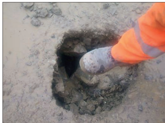
Figure 6. Small cavity on the 155m level, approximately above the location of the large open cave.
