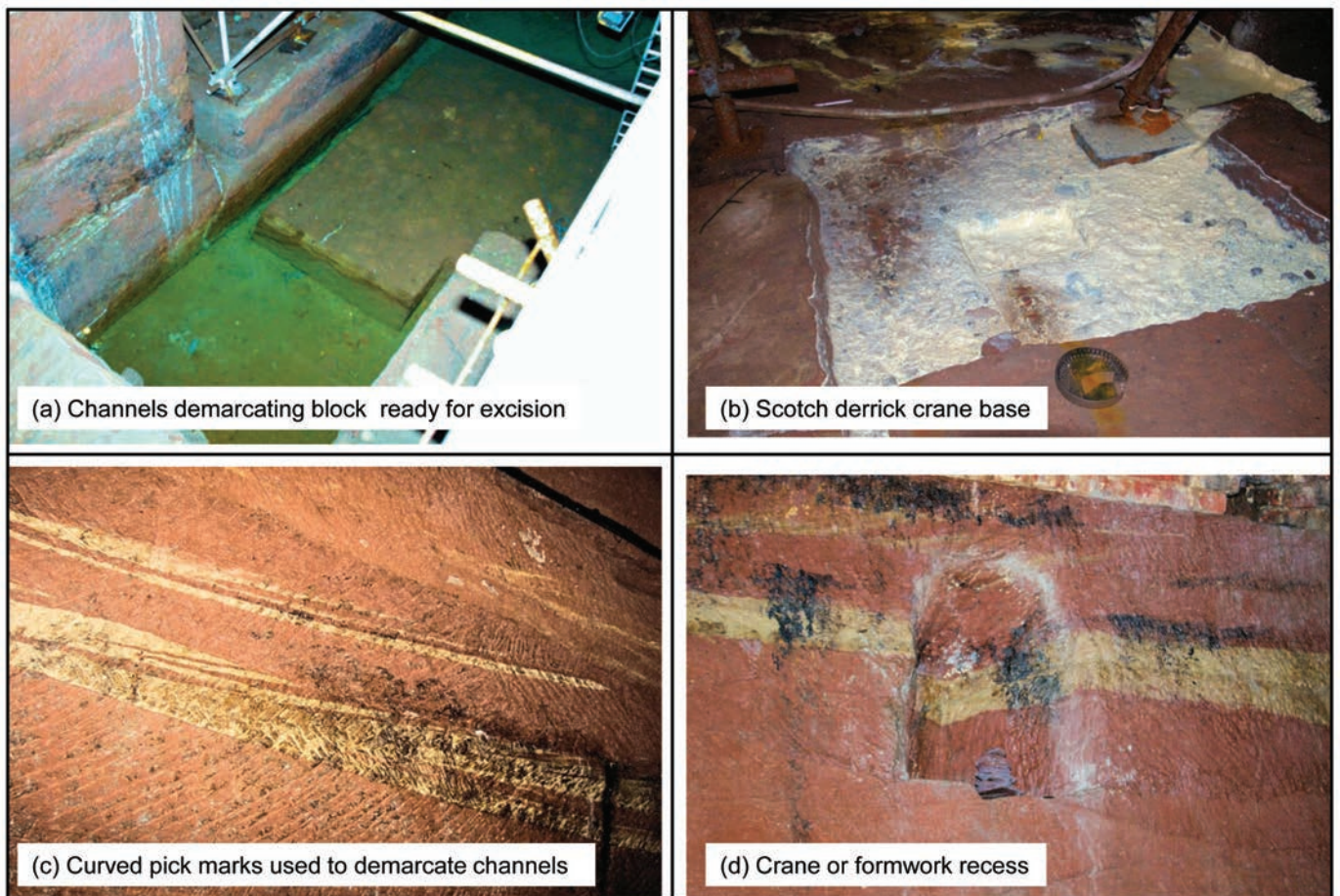
Figure 14. Building stone extraction features in the Williamson Tunnels Heritage Centre, Liverpool.
