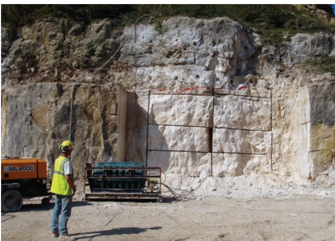
Figure 9. After cutting, the face has been sub-divided by a series of vertical and horizontal cuts into six discrete cantilevered blocks.
