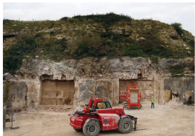
Figure 12. Oscillating (or place changing) the mining machine between the portals allowed it to cut continuously for maximum efficiency. It typically takes or 12 hours to cut a mine face which is the longest part of a production cycle.
