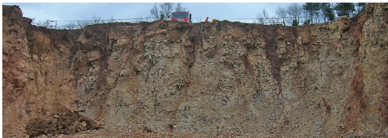
Figure 5. Box cut face showing broken rock clay with material infilling a number of fissures.
