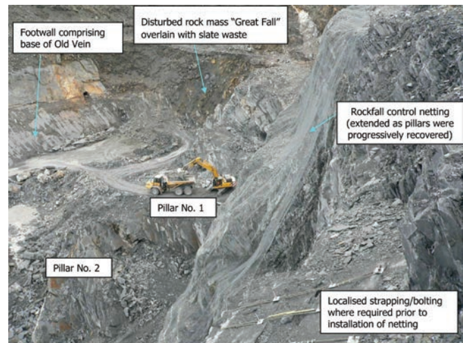
Figure 9. 2009-2010 development to recover Pillar No.s 1 to 5.
