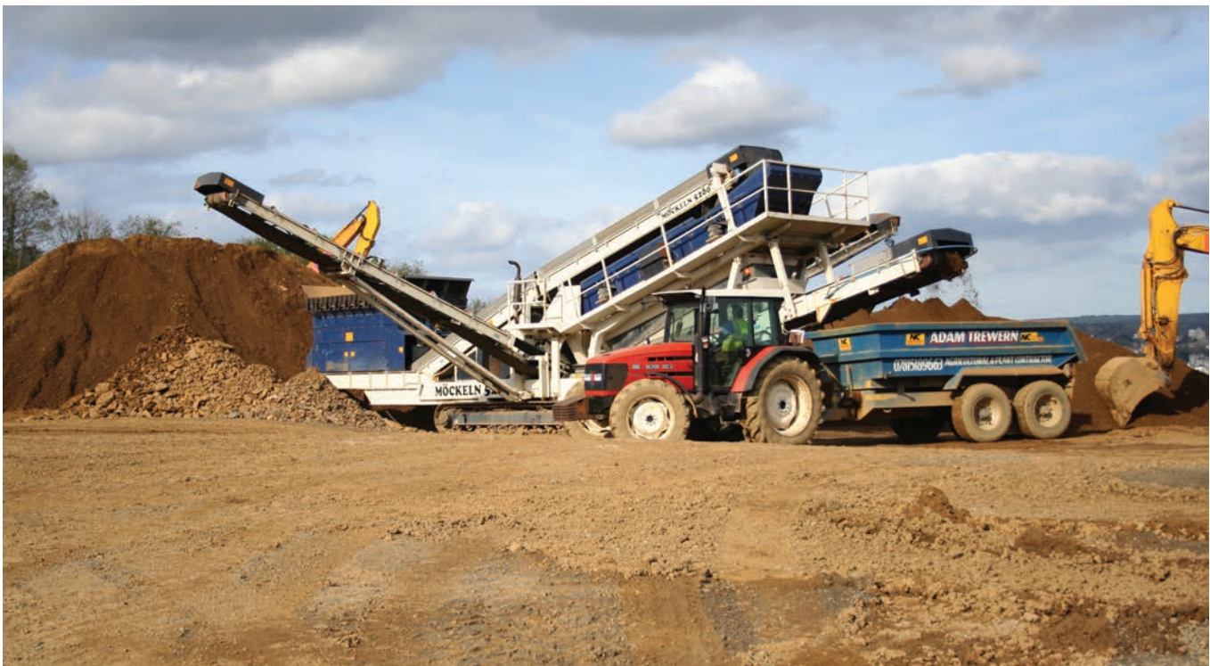
Figure 1. Re-processing quarry backfill at Penlee Quarry, Cornwall.
