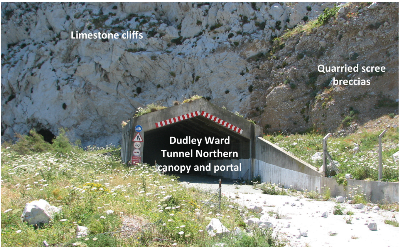
Figure 4. Original Dudley Ward Northern Approach tunnel portal.
