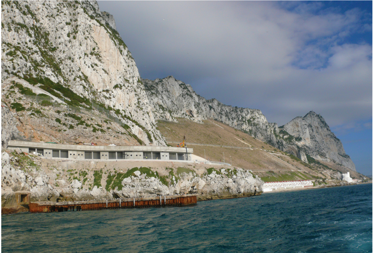
Figure 10. The completed 100m long rockfall canopy. Rock fall catch fences visible above the canopy. View looking northwest.
