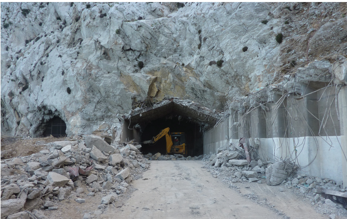
Figure 9. Demolition of the Dudley Ward Northern Approach old rock fall canopy.
