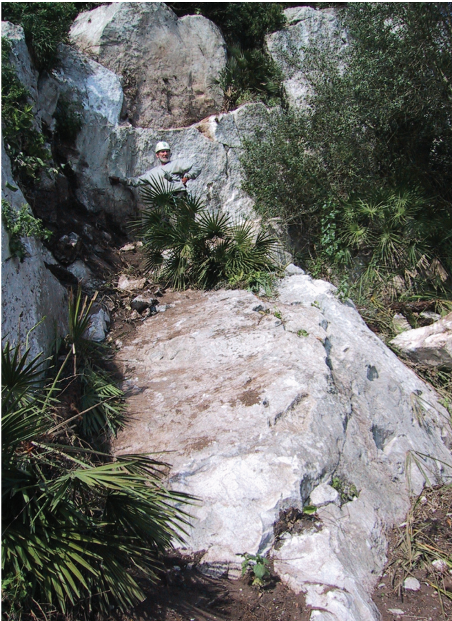
Figure 5. Location of the failed seeder block involved in the 2002 rockfall incident.
