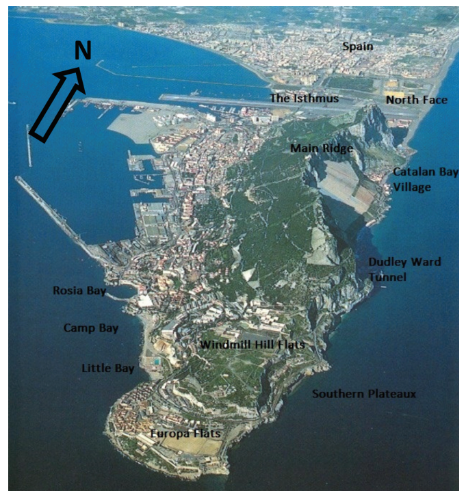
Figure 1. General view of Gibraltar, from the south.
