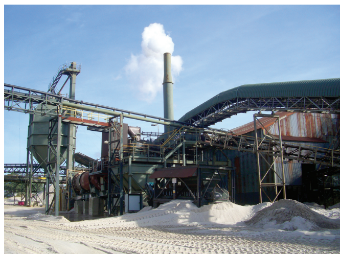
Figure 5. Silica sand processing plant, Norfolk. BGS © NERC
