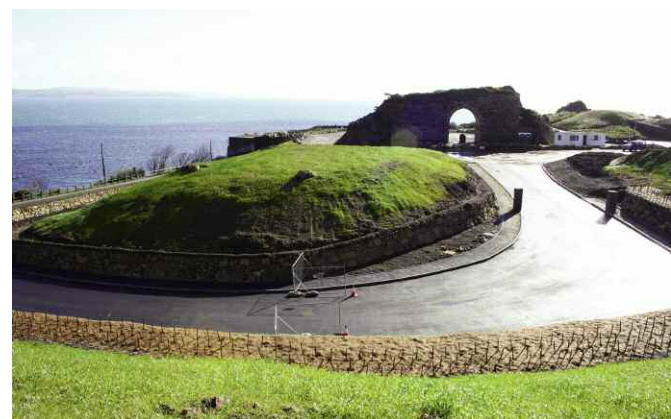
Figure 11. The new quarry entrance just prior to completion showing the archway that formerly carried the Newlyn – Paul road. The elevated ground in front and to the left of the archway comprises mainly metadolerite whereas the road runs through former quarry backfill.
