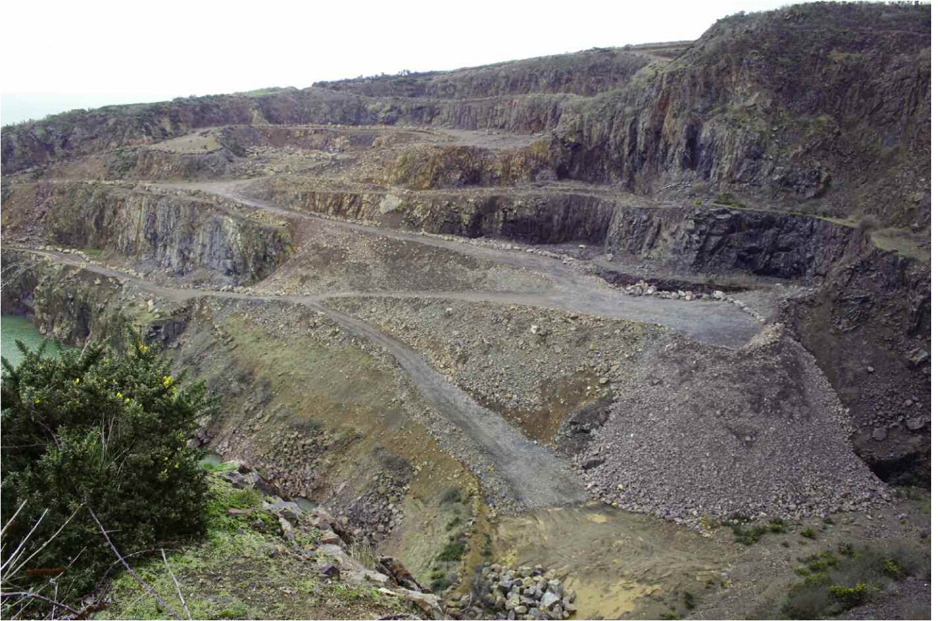
Figure 12. A general view of the proposed armourstone quarry benches looking SSE immediately after the removal of unexploded explosives.
