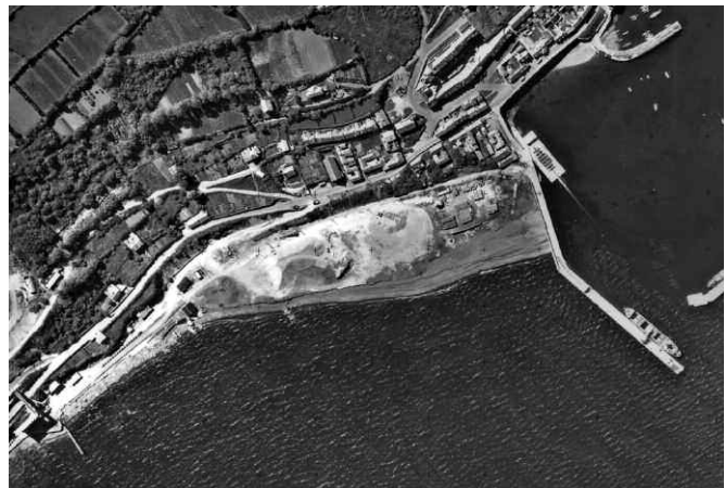
Figure 8. An aerial view of the main shipping arrangements for the export of aggregate circa 1970 showing two trains carrying tubs to a vessel at Newlyn south pier. The local road network includes several pinch points with road widths of less than 4.5m compounding export problems.
