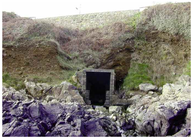
Figure 7. The 1948 adit used for discharging surface water collecting in the workings. This adit passes under the Newlyn – Mousehole road onto the foreshore. The adit lies near the proposed breakthrough to the sea.
